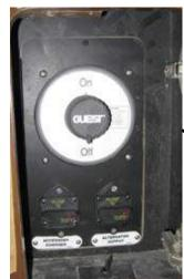
Electricity from the battery to the Safety Breaker Panel is controlled by a master disconnect switch. This switch is located in a cabinet in the starboard side of the salon. To provide electricity to the Safety Breaker Panel, turn the master disconnect switch to the ON position. Circuit breakers on the Safety Breaker Panel control the other DC circuit breaker panels.
