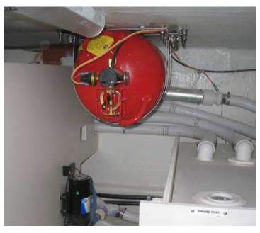
A fire suppression system monitor, installed near the helm, is wired to an ignition switch. The monitor's light should be ON when the ignition switch is turned ON.
