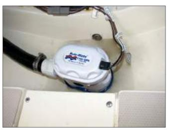
Bilge Pump W/ Built In Automatic Switch In Aft Systems Compartment
