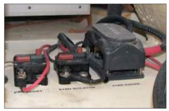
Typical Yamaha Engine Charging Circuit & Power Assist Steering Heavy Duty Circuit Breakers
